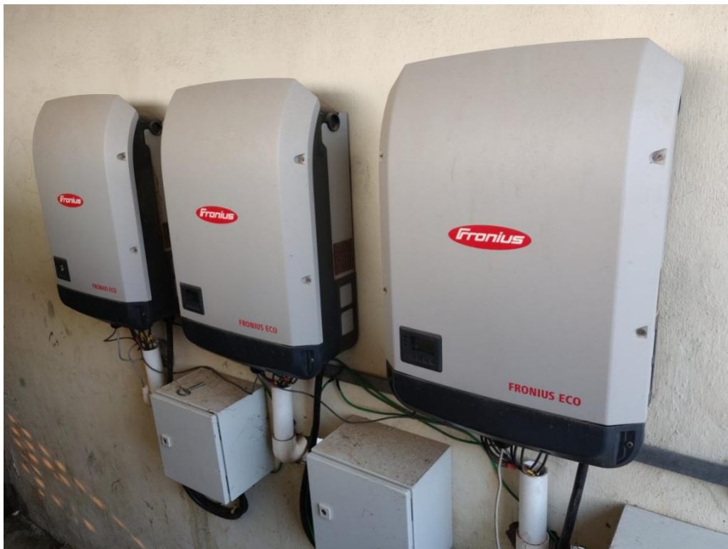
Grid-Tie inverters connected to 100kWp Solar PV Plant. Solar PV Energy Generation Reports for the Year 2018.
