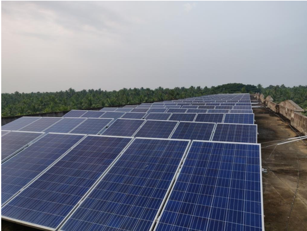
Solar PV Plant - 100kWp installed on Administration block
